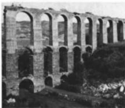
PLATE 19.3 Aqueduct from Zaghouan, which supplied Carthage
