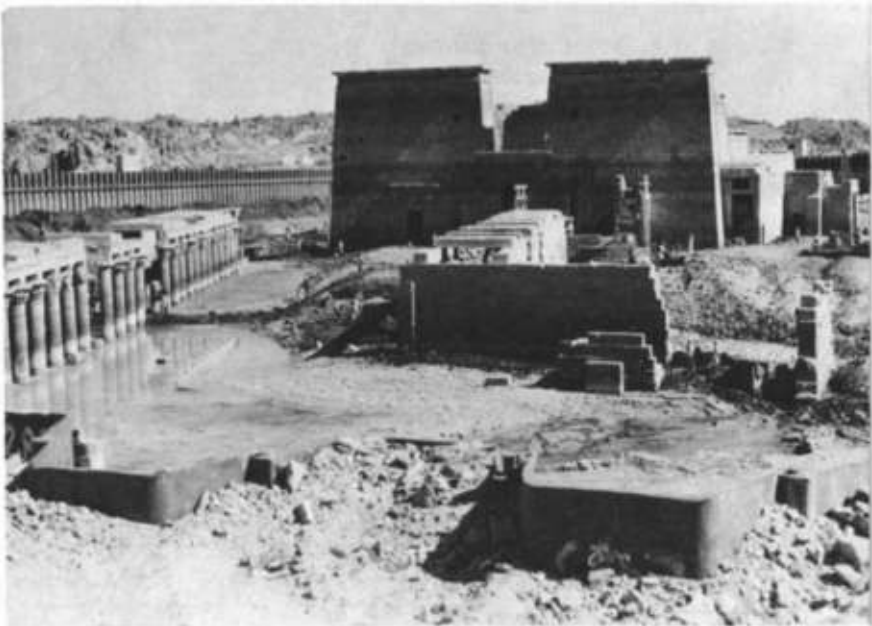
PLATE 8.1 Nubian monuments of Philae being re-erected on the neighbouring island of Agilkia
